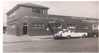
▲ The original G&H Chemical Industries building.
