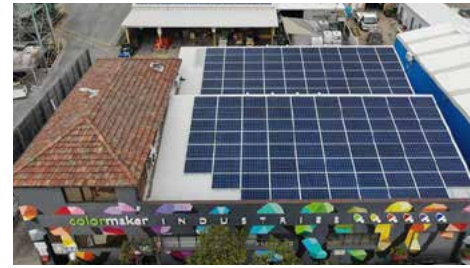
Colormaker Industries' rooftop powerhouse
