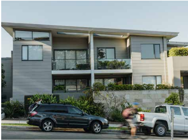
Multi-dwelling housing, Manly
